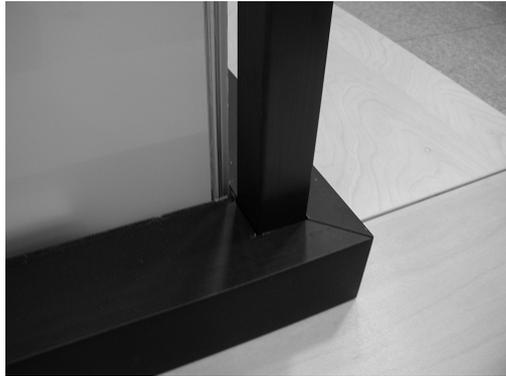
**Figure 7.2** Support frame with vertical reinforcement and glass panels installed
